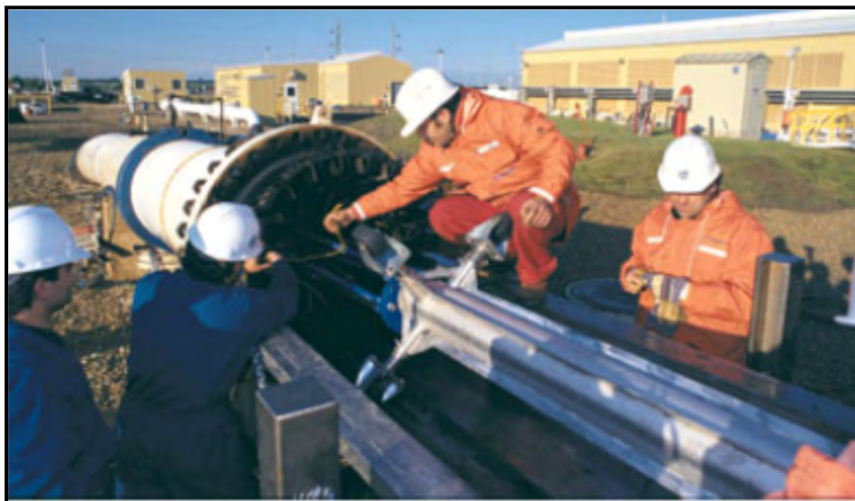
Figure 4-14 Crew inserting pig into natural gas supply line at pigging station
