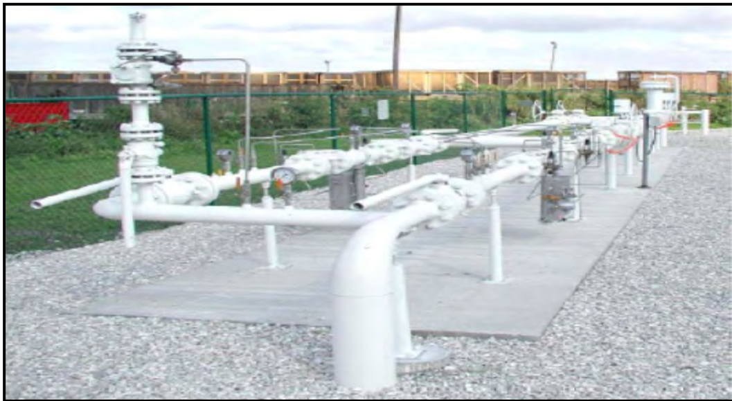
Figure 4-12 Typical city gate station (similar to proposed connection near Sand Hollow)
