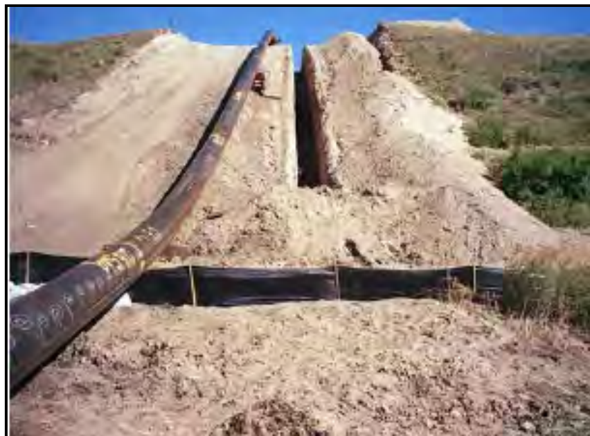
Figure 4-10 Typical installation of natural gas supply line
