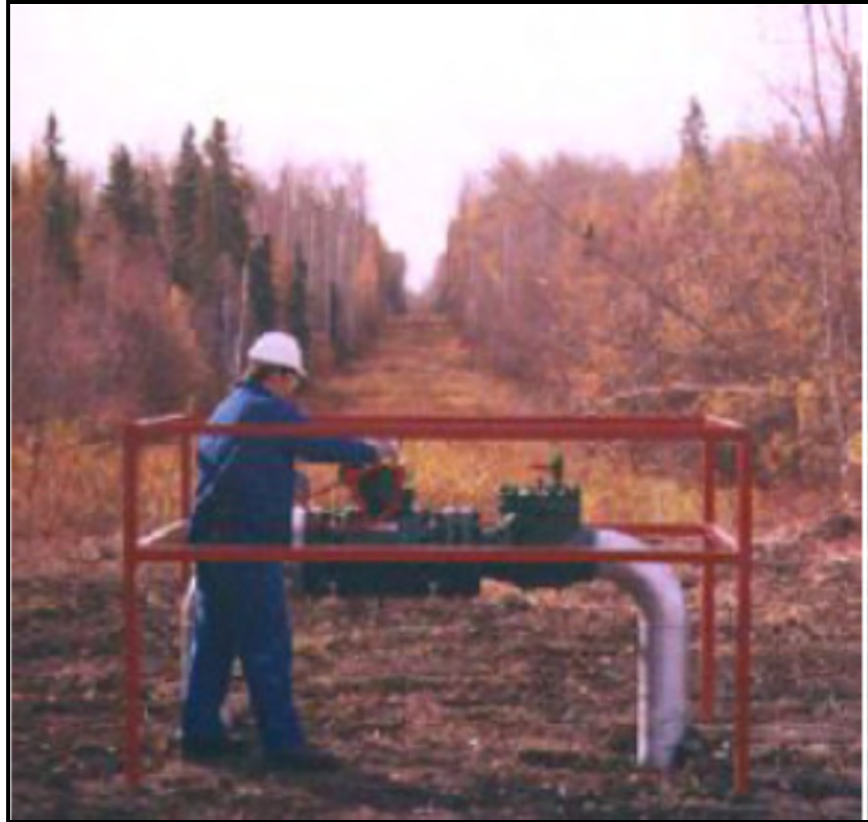
Figure 4-13 Typical aboveground valve on natural gas supply line
